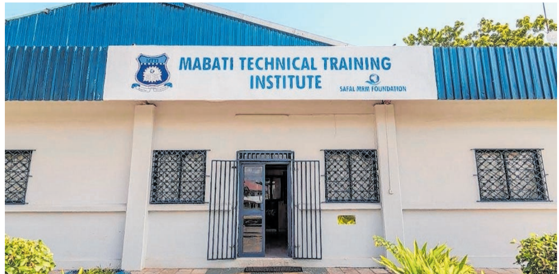
Mabati Technical Training Institute; a training facility by Mabati Rolling Mills in Mariakani Kilifi county to ensure quality products from the organization.
